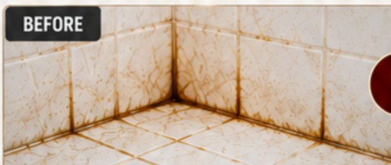
RUST-STAINED TILE SURFACE
